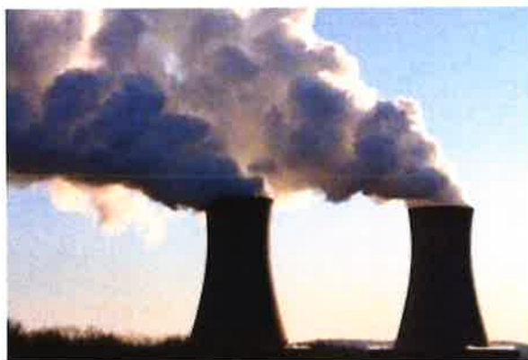
Limerick Nuclear Power Station
