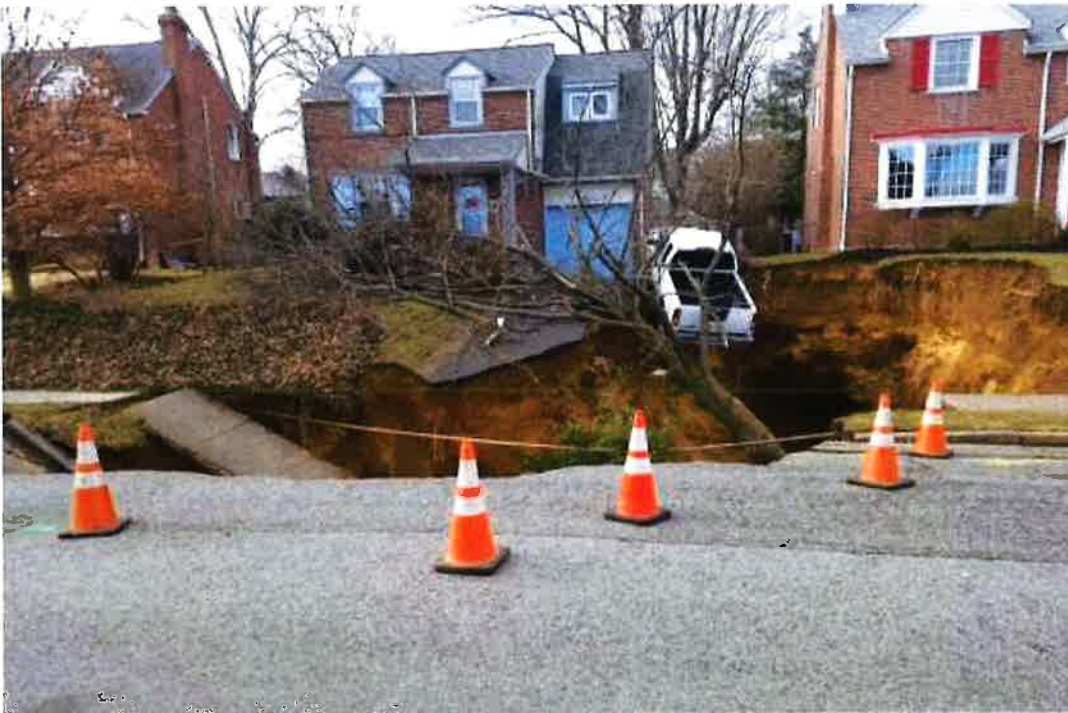
Sinkhole at 720 and 724 Brooke Road
