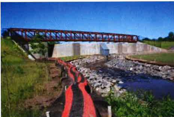
Flood control structure in Upper Dublin Township
