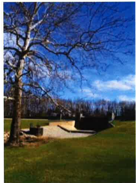
Loch Alsh Dam spillway
