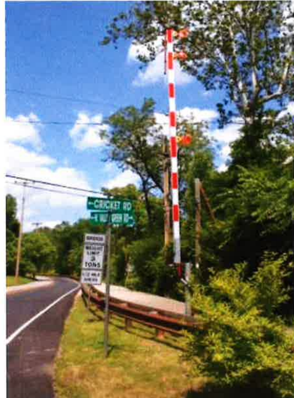
Flood warning gates in Whitmarsh Township
