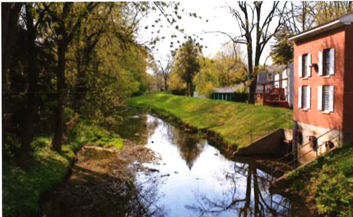
Stormwater pump station on the Tookany Creek
